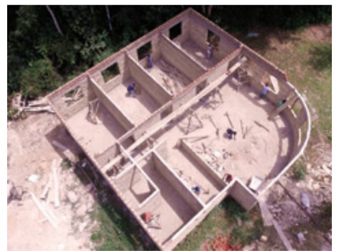
▲ The next Family Unit is being built
